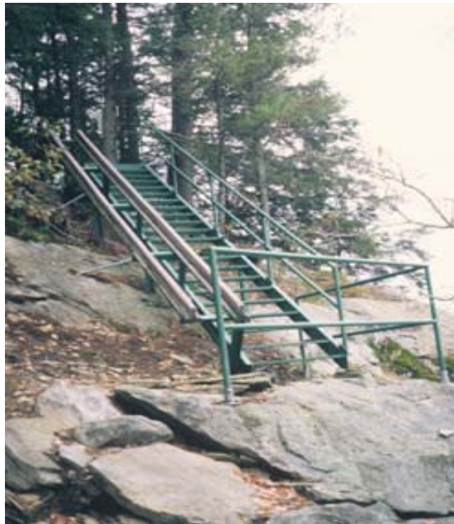
Photo 10E: Metal staircase with boat slide facilitates river access from a steep, rocky shoreline
