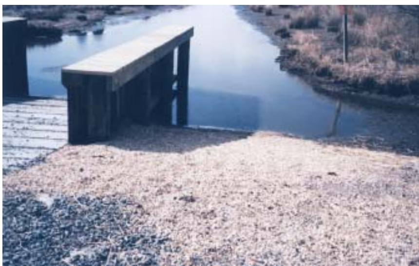
Photos 11B: Geocell material anchored with pea gravel offers low-impact access while helping to stabilize an eroding bank
