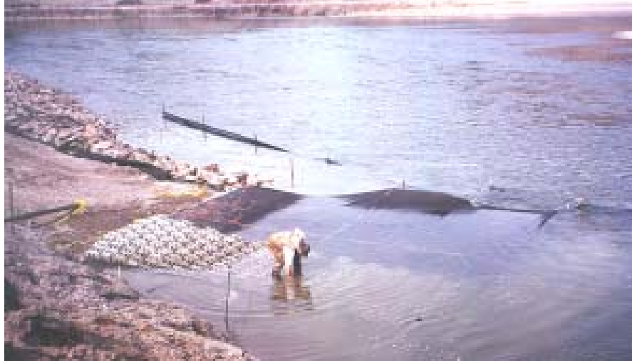
Photo 8J: Concrete mats are installed individually
