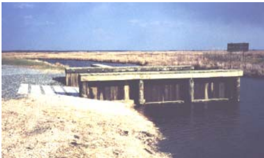
Photo 11A: Geocell material provides paddlers with a “soft” launching alternative to a traditional boat launch
