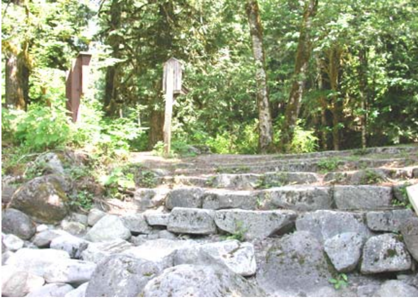
Photos 9F, 9G: Rock staircase provides river access with a “natural” appearance
