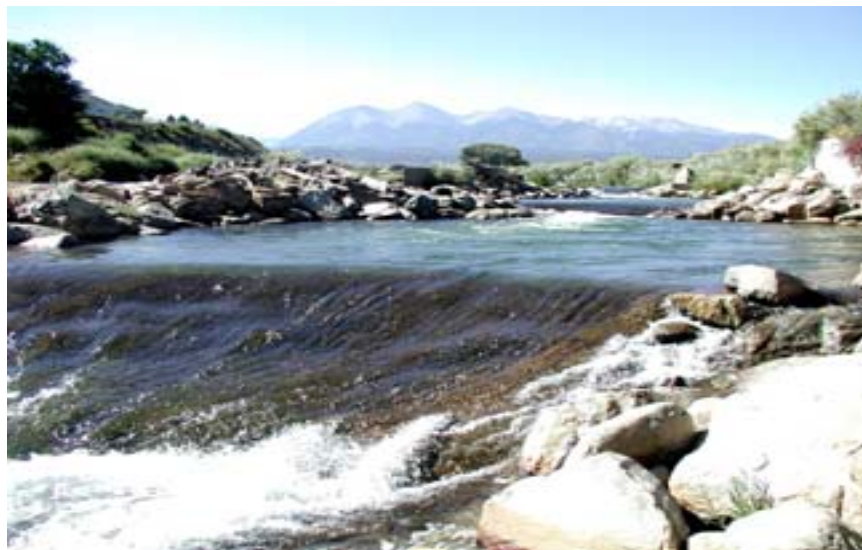
Photo 10K: Whitewater chute, installed just east of dam, offers paddlers rapids on three 2' drops
